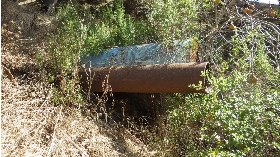
Photo 3. Shotgunned Culvert 3 outlets.
