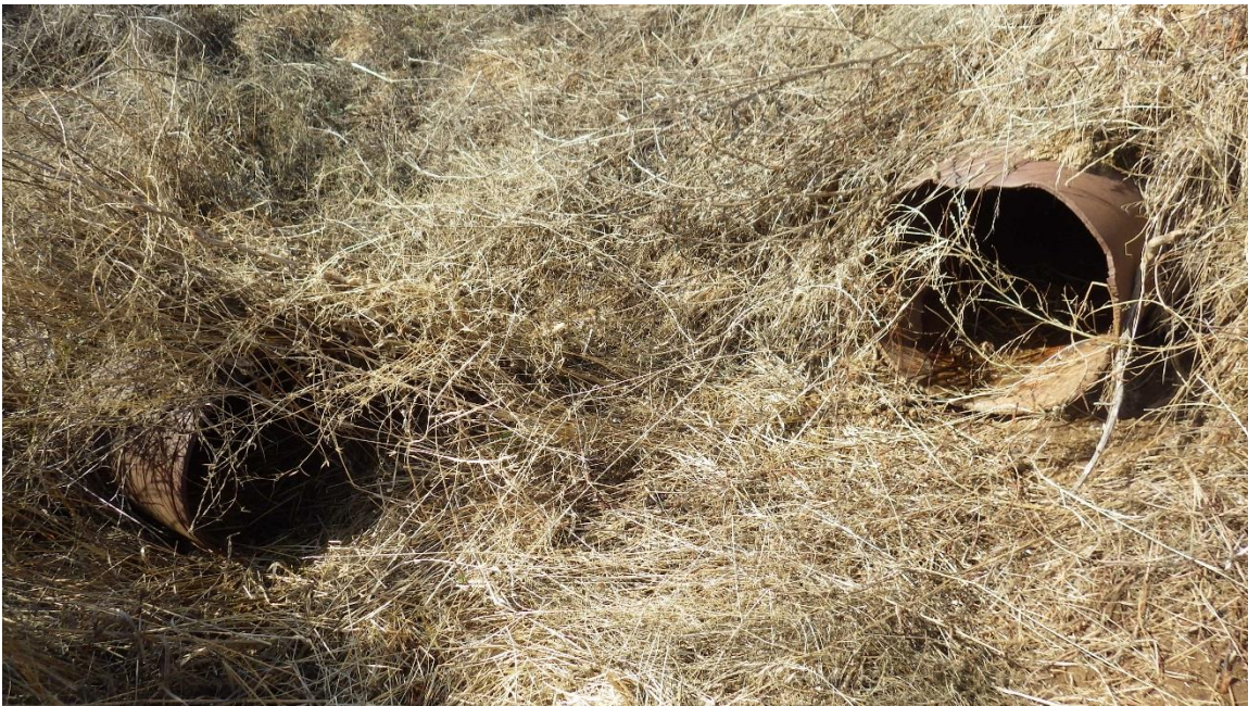
Photo 6. Culvert 5 outlet and Culvert 6 inlet. Culvert 5 inlet completely buried with sediment.
