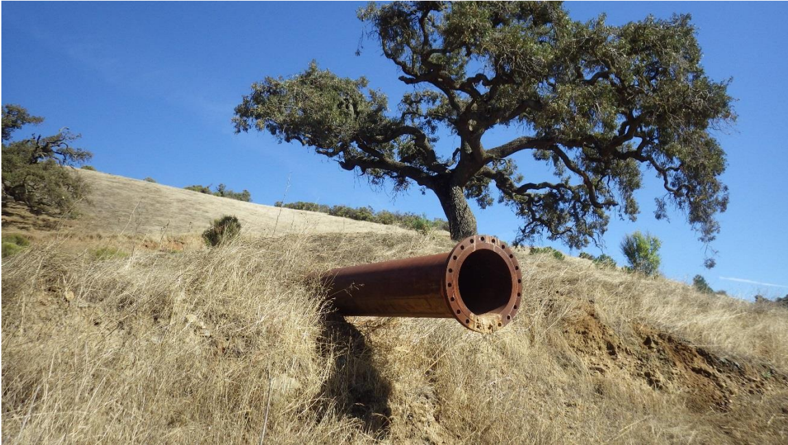
Photo 7. Shotgunned Culvert 6 outlet.
