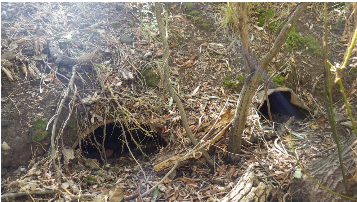
Photo 4. Clogged Culvert 4 inlets.
