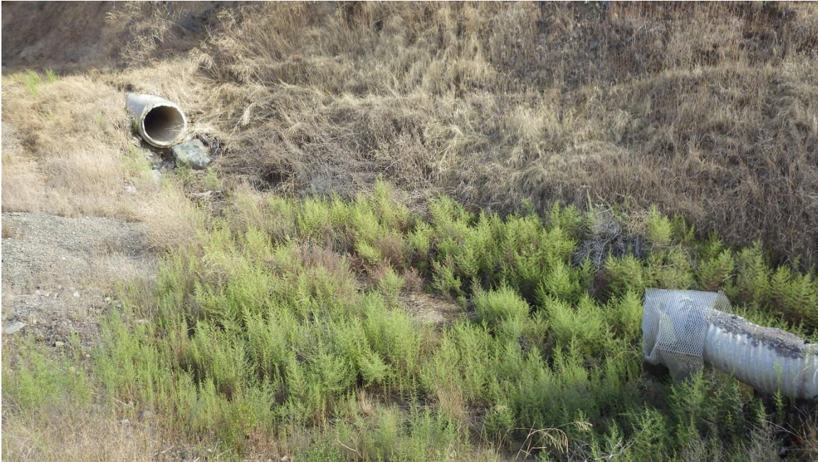
Photo 1. Outlet of Culvert 1 (top of photo), catchment basin, and inlet of Culvert 2 (bottom of photo). Evidence of clogging of Culvert 2 inlet in the form of sediment on top of culvert and heavy equipment bucket tooth marks on culvert.
