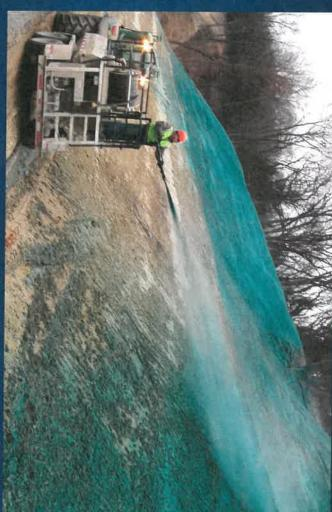
Once stockpiles of dirt are complete, they are treated with a hydroseed to vegetate the slope with grasses, controlling dust and erosion.
